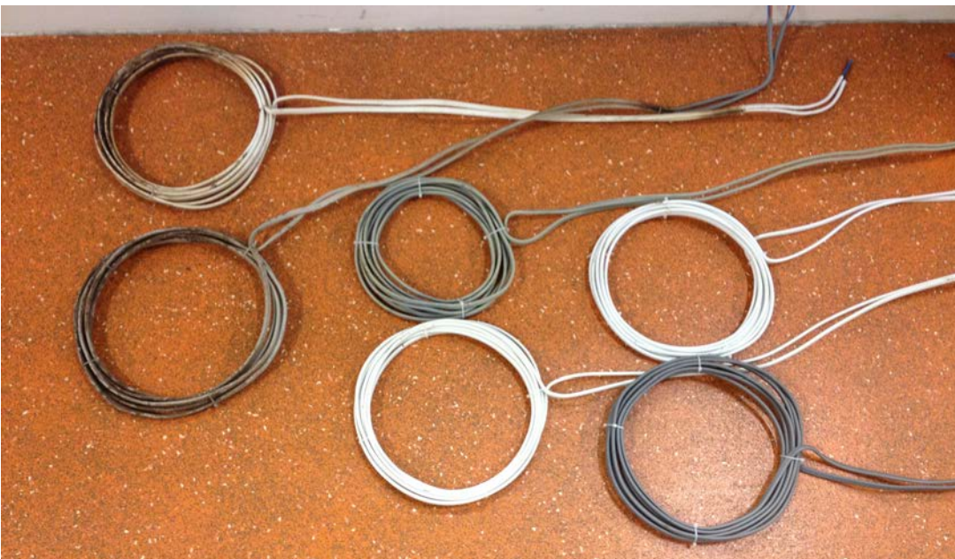
Figure 4: Condition of cables after Protocol 4 – Medium Term Immersion Insulation Resistance. Left to right: silty, salty, clean. Grey cables: PVC; white cable: LSHF.
